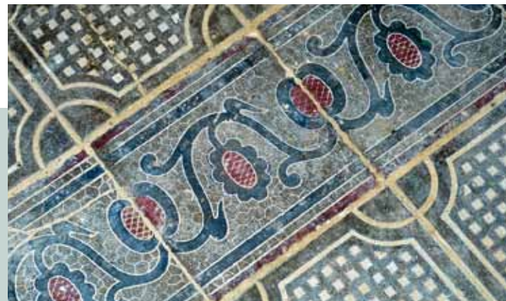
Hallway tiling detail
