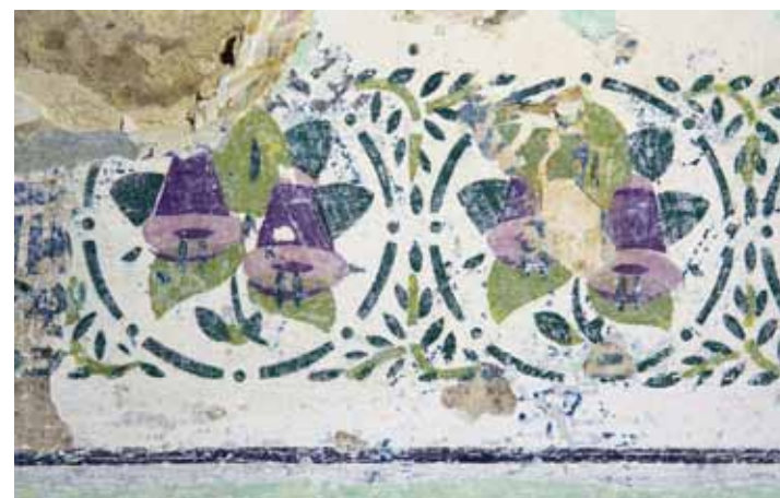
Detail of stencil painting on the interior walls
