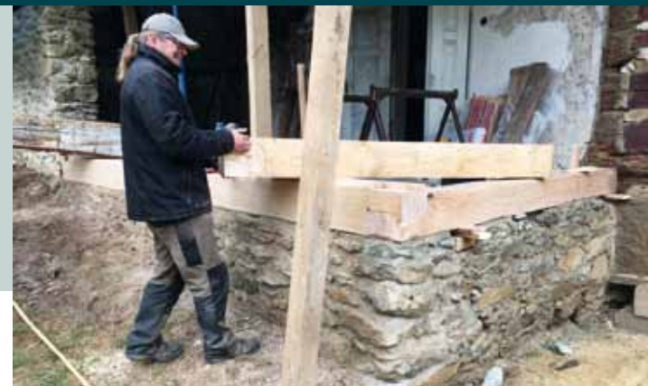
Skilled carpenter Tomáš Kracík at work
