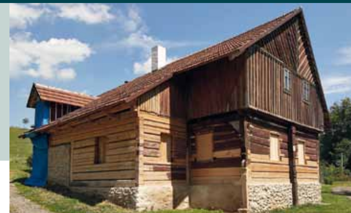
State of renovation in June 2017
