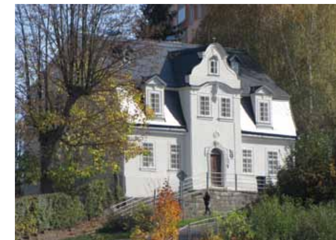
Current state of the house after the latest extensive renovation in 2017.
