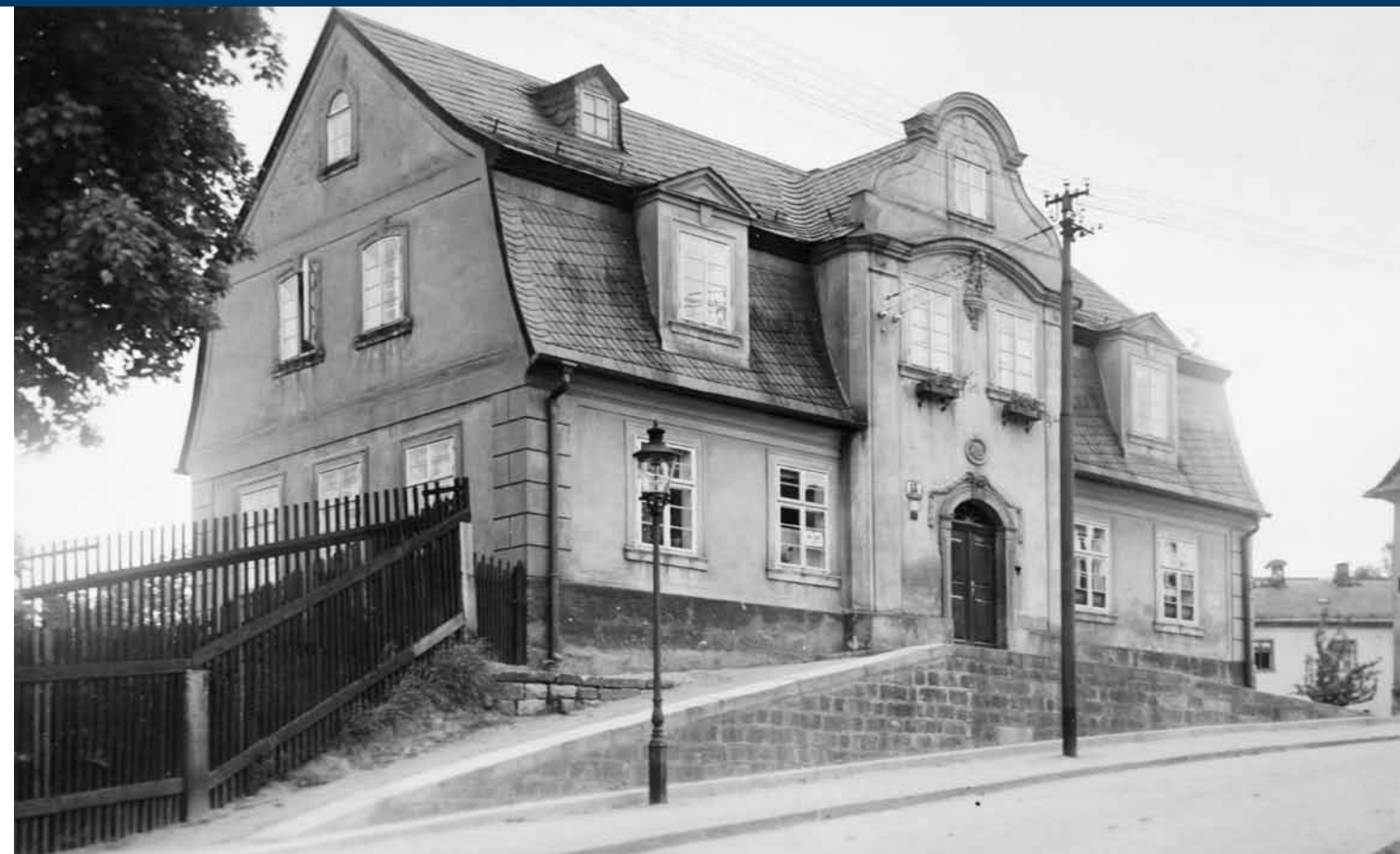
Photo from the early 1930s showing the original slate roof.
