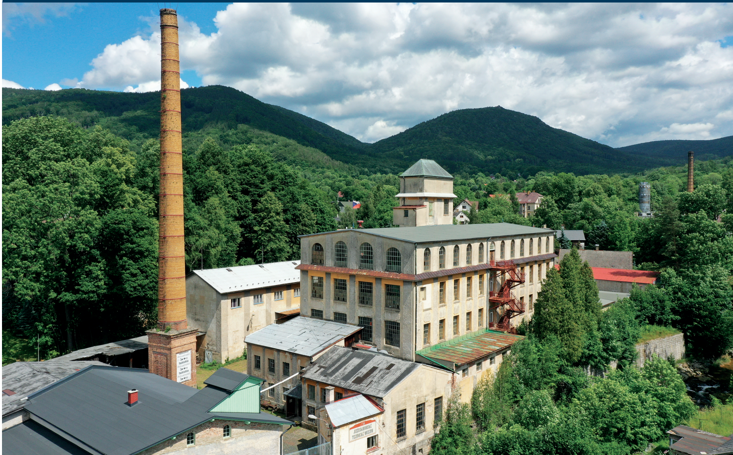
General view of the spinning mill area from the west
